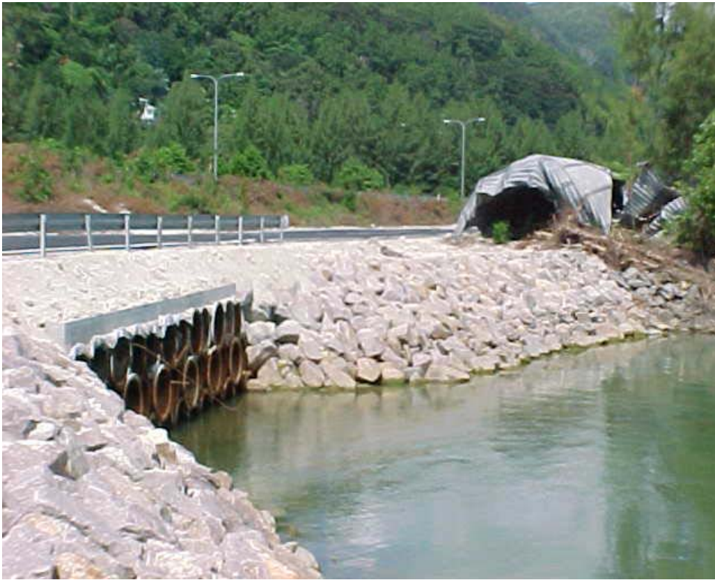
Plate 3: Temporary repairs on Roche Caiman Bridge
